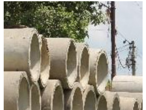
Figure 31: STP construction and laying of underground sewer line in progress
