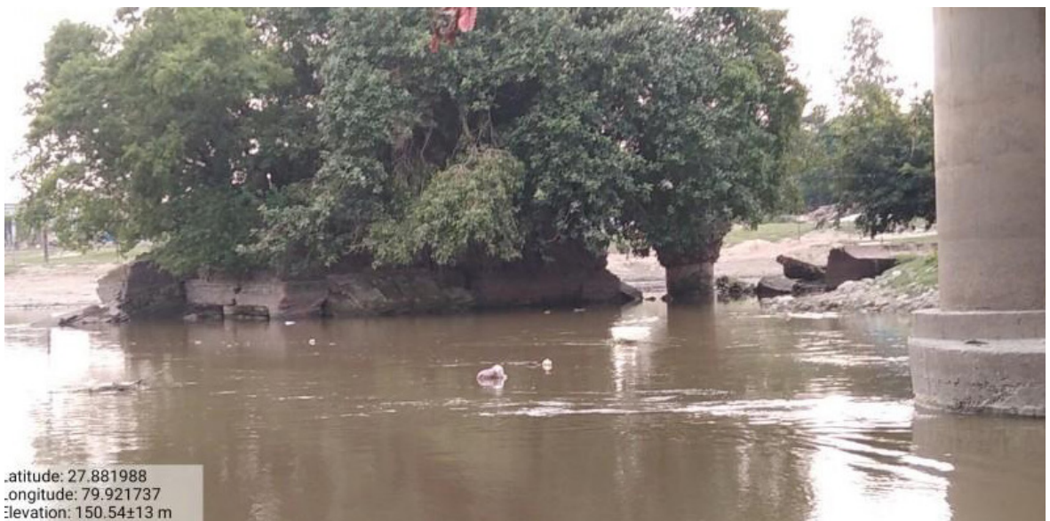
Figure 33: Debris of old Lodhipur bridge
