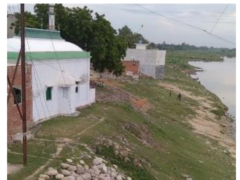
Figure 27: Encroachment on Garra river near Aziz Nagar Bridge
